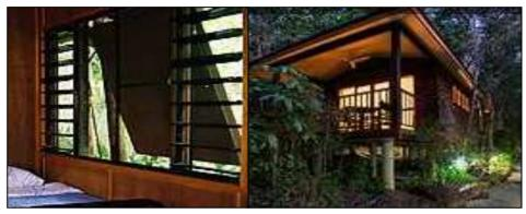
Example of awnings comprised of timber battens to encourage shade and protect openings (*Images sourced from:* <u>http://www.thalabeach.com.au/port-douglas-accommodation/</u>
