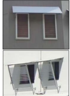
An example of louvres that are designed for tropical climates being shaded by an awning
